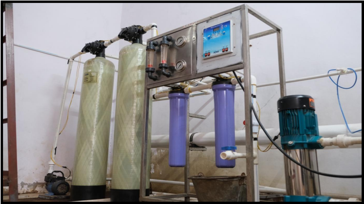
PURIFIED RO WATER PLANT IN COLLEGE CAMPUS WITH 4000 LTRS CAPACITY IN CAMPUS
