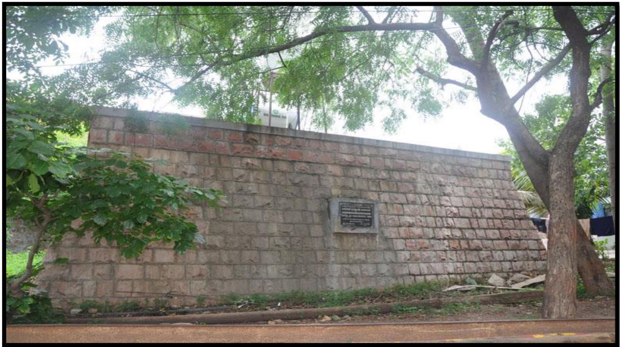
WATER STORAGE TANK FOR LADIES HOSTEL
