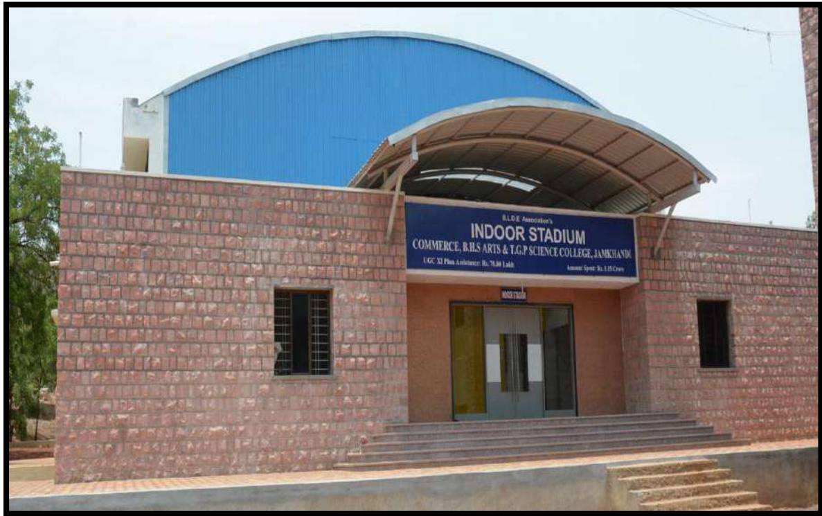
FRONT VIEW OF INDOOR STADIUM
