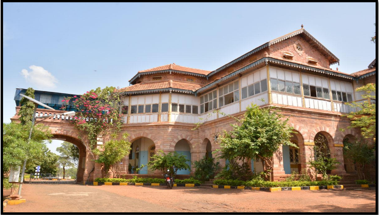
OLD ADMINISTRATIVE BLOCK
