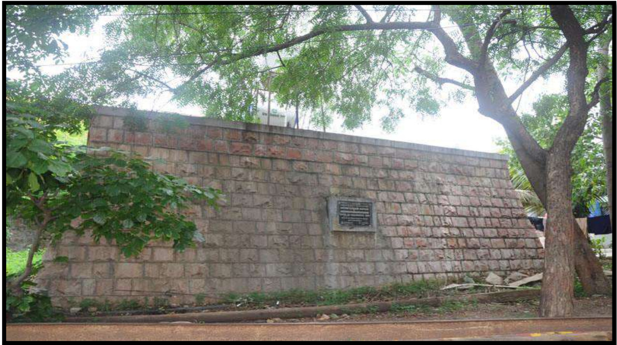
WATER STORAGE TANK FOR LADIES HOSTEL
