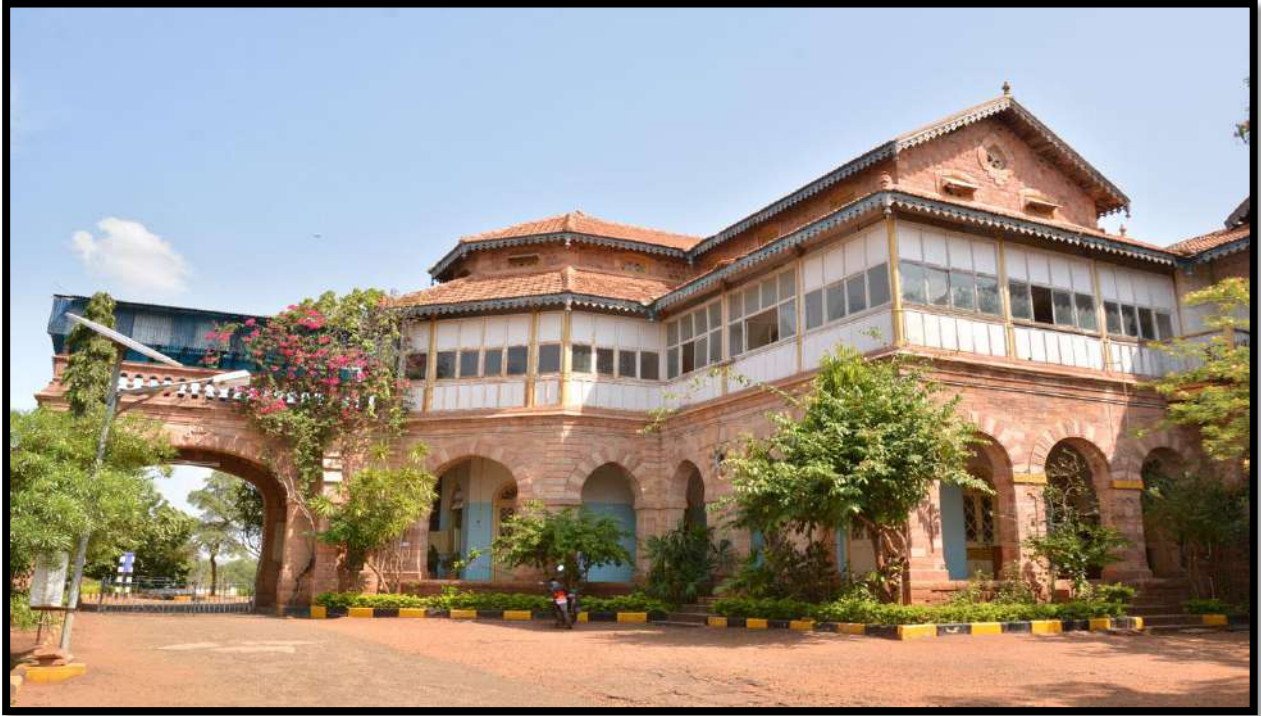
OLD ADMINISTRATIVE BLOCK
